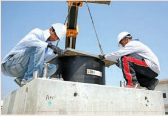
Base isolators being fitted
