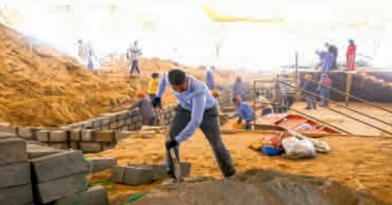
Excavating and reinforcing the shilanyas foundation area
